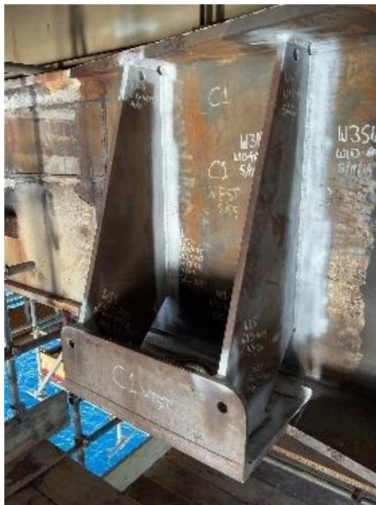
One of the lift points installed on the Fortescue facility
