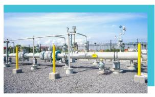
The GtE pipeline is the first natural gas pipeline in Guyana. It will operate at high pressures (above 1,800 pounds per square inch (psi) or 12,400 Kilopascals (kPa)).
