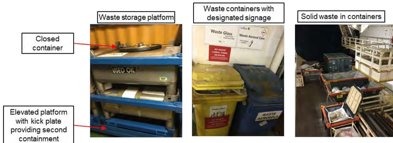
Each maritime vessel has designated waste storage areas, and these waste storage areas are often on multiple decks to facilitate operations. As per the MARPOL 73/78 and IMDG requirements, each vessel is required to have pollution control measures that are related to all operations, including waste storage operations.
